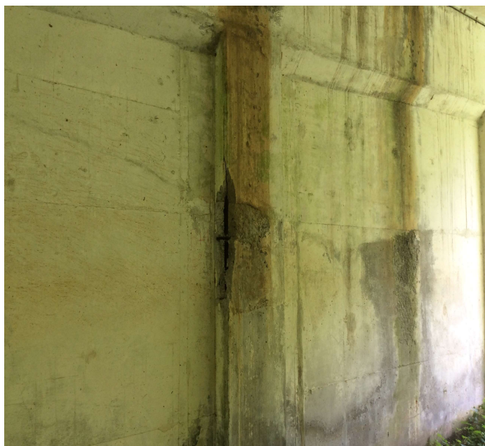
PHOTO 3 Description Bent 4, Column 2 has a 3' long spall with exposed reinforcing steel with initial section loss.
