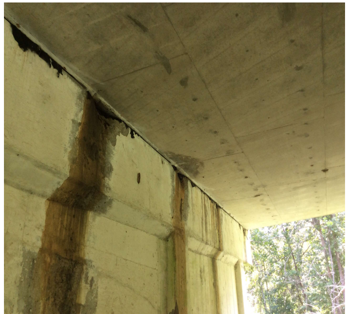
PHOTO 2 Description Bents 2, 3 & 4 have concrete spalling with exposed reinforcing steel at the keyways. Bent 3 pictured.
