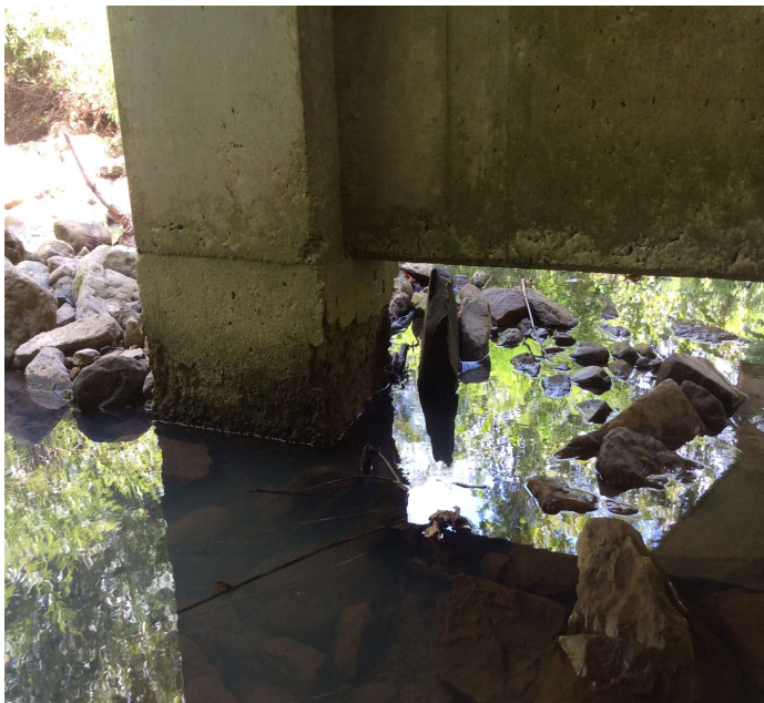
PHOTO 1 Description Concrete spalling and deterioration at the base of Bent 2, Column 1 with no exposed reinforcing steel.
