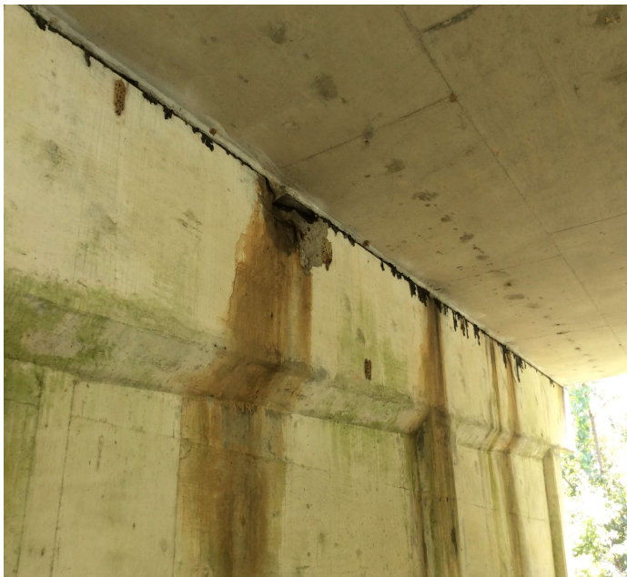
PHOTO 1 Description Bents 2, 3 & 4 have concrete spalling with exposed reinforcing steel at the keyways. Bent 2 pictured.
