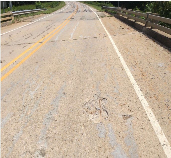
PHOTO 1 Description Span 3 Rt lane has a 2' x 1' spalled area with exposed reinforcing steel in the wheel path.
